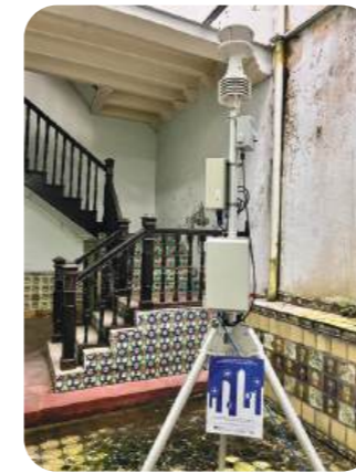
Weather station that monitors air flow, humidity, temperature, solar radiation and air pollution concentration.
