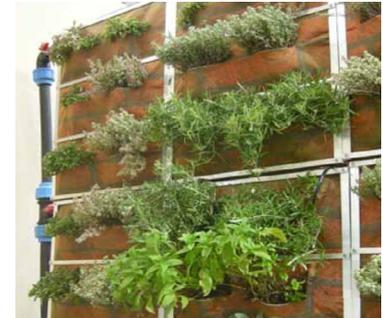
**Fig. 5** Green wall with layer for cultivation
