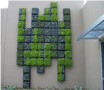
**Fig. 3** Panel with soil substrate cells for planting
