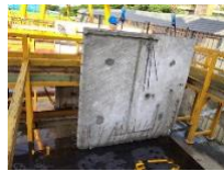
2D Precast Panel Assembly Preparation
