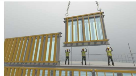
Figure 21 Vertical fins are prefabricated as part of the precast wall
